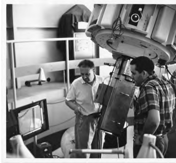
Photo 11. Kuiper and engineer Richard Goranson with the IR spectrometer on the Kitt Peak 36-inch telescope during daylight observations, 1962. Photo by D. Cruikshank
