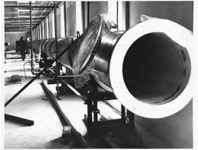
Photos 15 and 16. Photo 15 shows graduate student Toby Owen with the small (62-ft) absorption cell in the original Lunar and Planetary Lab facility. He used data obtained with that tube for his dissertation on planetary spectroscopy (LPL Photo). Photo 16 shows the larger 40-m absorption cell under construction in the new Lunar and Planetary Laboratory (now the Kuiper Building). Photo by D. Cruikshank
